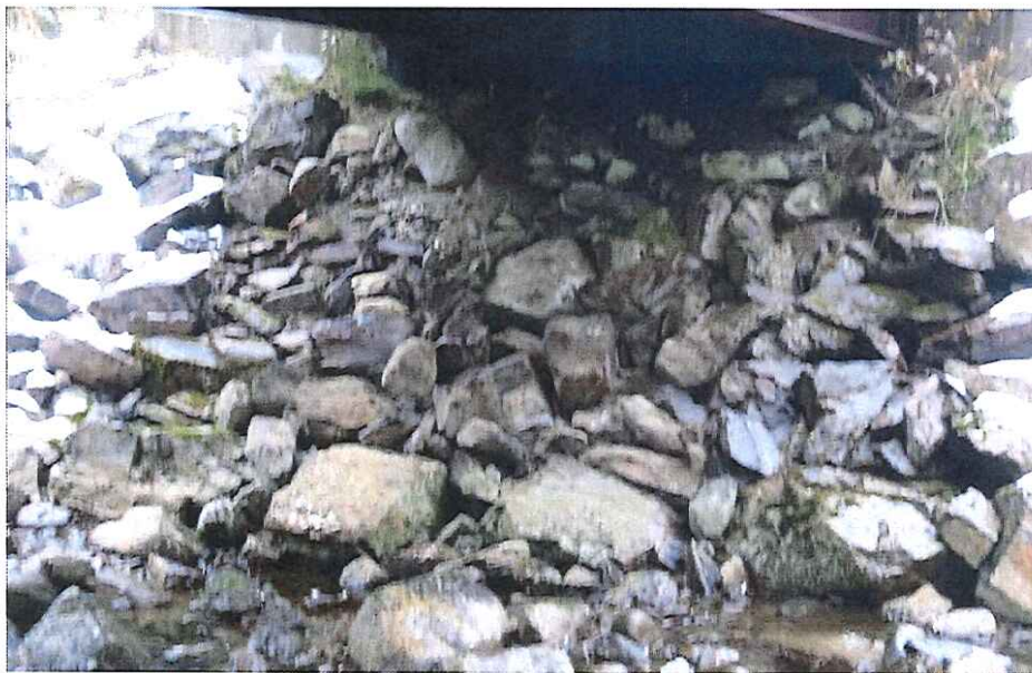
CK2317 Right Abutment
