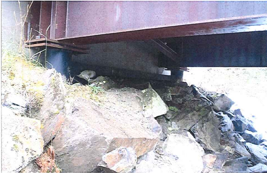
CK2317 Left Abutment
