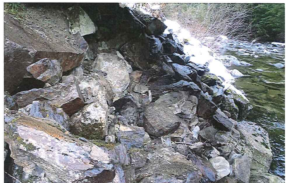
CK2317 Left Abutment riprap
